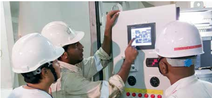
Blue Ocean Solutions Senior Engineer, Mr Thomas Tesswin (second from left), explaining some of the functions of the EFS Water Controller to APL crew members
